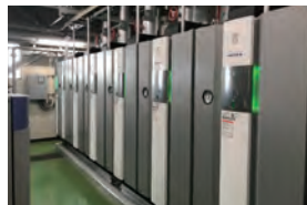
Once-through boilers at the Urawa Factory
